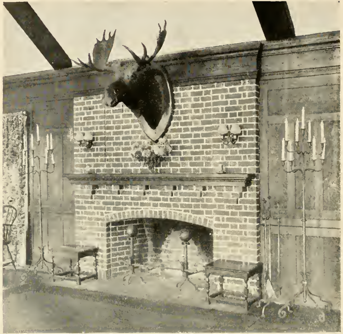
A Great Brick Fireplace with Seats on Either Side
